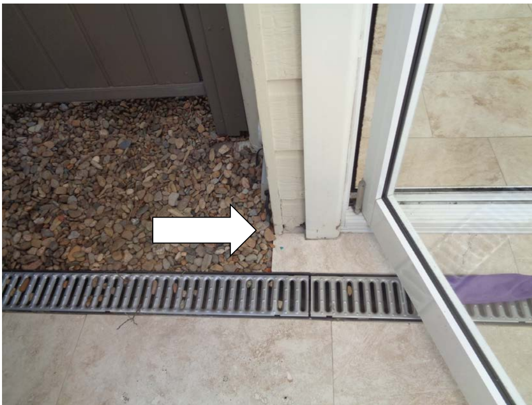
Damaged cladding
