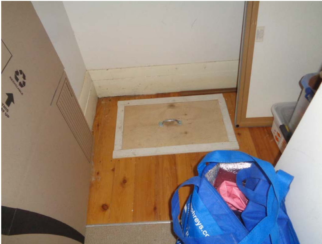
Man hole access to subfloor
